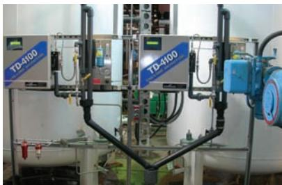
TD-4100 fluorescence oil-in-water monitors protecting power plant lake intake from oil spill contamination in Alberta, Canada.
