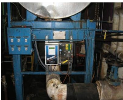
TD-1000C fluorescence oil-in-water monitor protecting boiler feed water from oil contamination.
